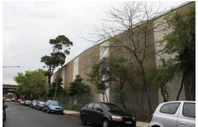
Figure 7: Looking west along the Macdonald Street frontage of the site
