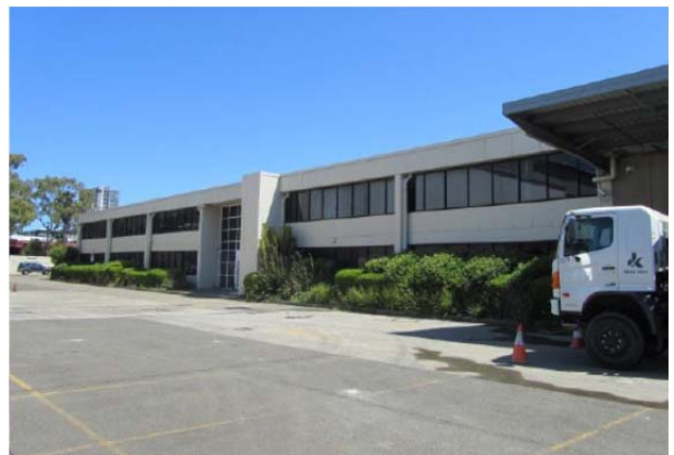
Figure 9: Eastern elevation of warehouse showing attached office
