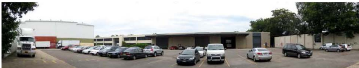
Figure 3: View of site (pre-demolition)
