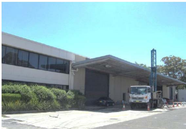
Figure 8: Eastern elevation of warehouse with part view of attached office building
